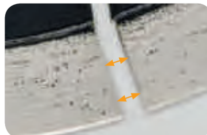
The vibration load can be minimised thanks to more uniform narrow gaps between the segments.
